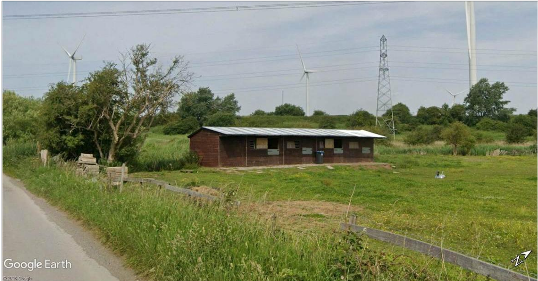
Figure J89 View towards the reflecting panels from Moorditch Lane - Google Streetview
